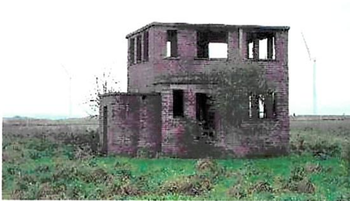
The remains of the Control Tower built during WWII
