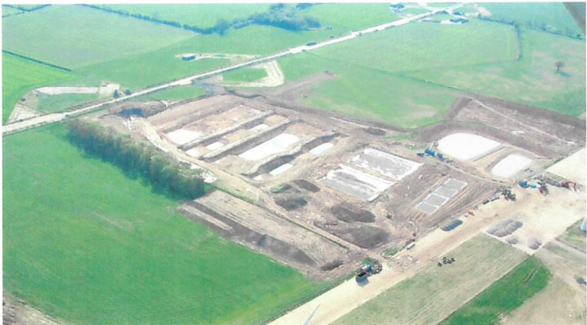
An aerial view of the reed beds under construction
